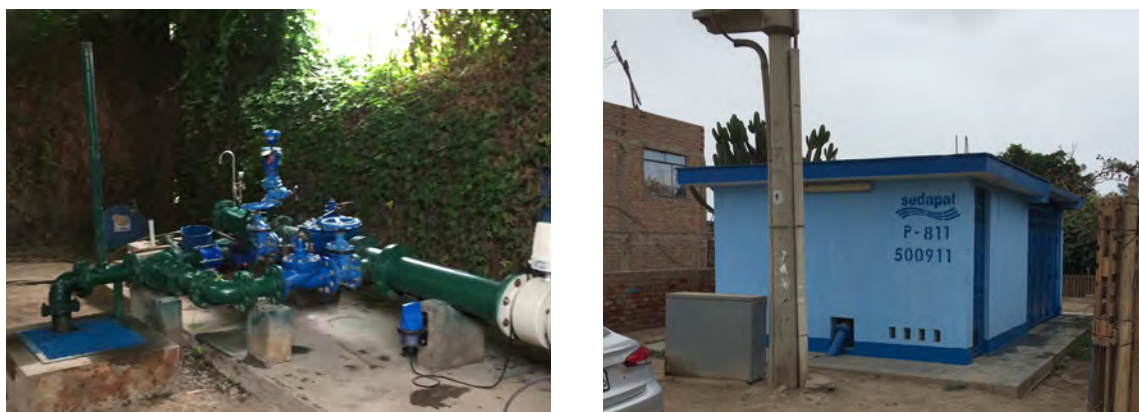
» Figure 5.4: Well head (left) and well building (right) of a SEDAPAL well. Pictures: S. Stauder.
