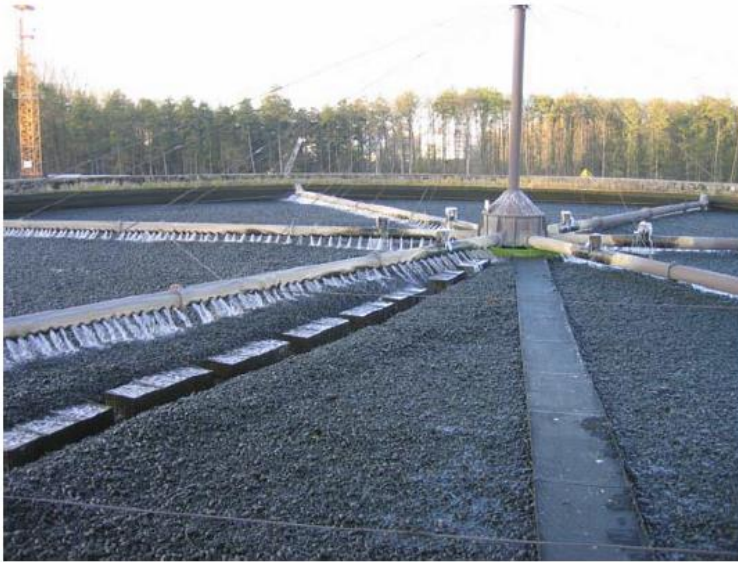
Topview of a trickling filter filled with lava rocks (Sindelfingen, Germany)
