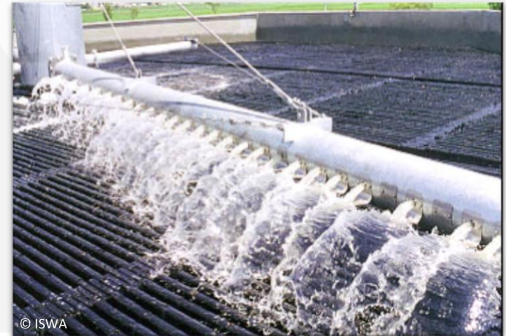
Topview of a trickling filter with plastic profiles
